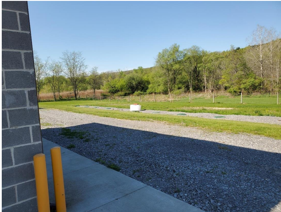
Figure 2: Photo of Buried Septic Tanks
