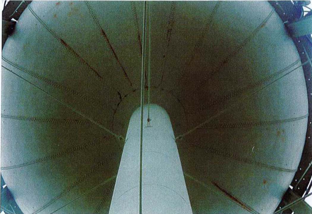
Photo shows the condition of the riser pipe and bowl connection, which appears to be in good condition.
