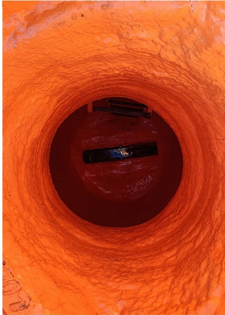
MH Lining Completed January 2024
