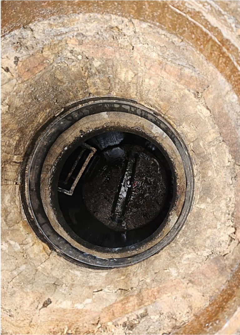
Signs of Infiltration at MH barrel and bench, along with deterioration of structure
