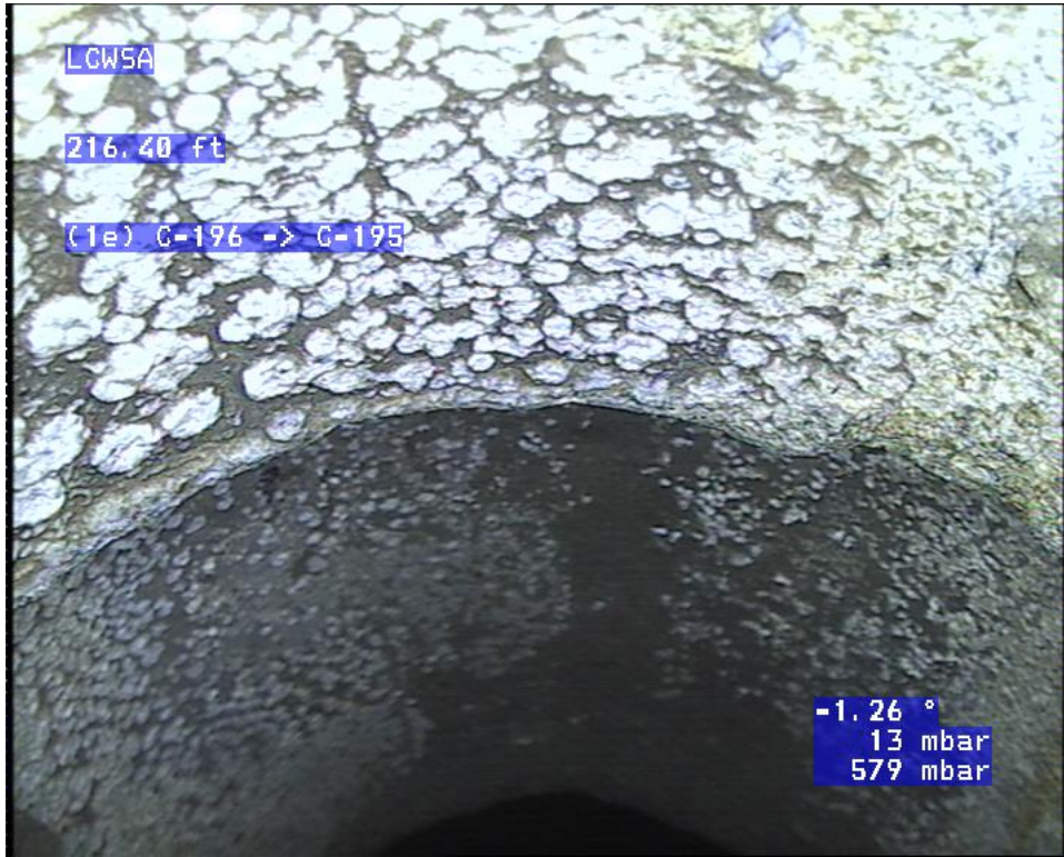
Pictured above and below: 8" ACP sewer main downstream of PS 1E is very pitted and corrosion is evident.
