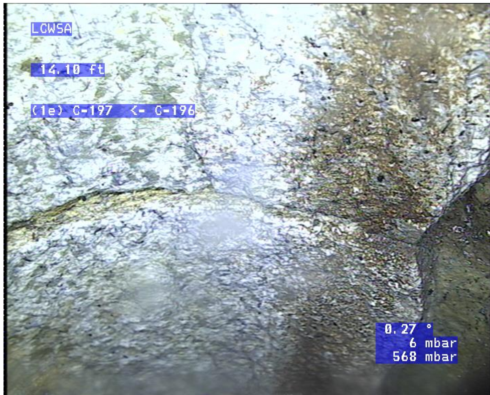
Pictured above and below: 8" ACP sewer main downstream of PS 1E is very pitted and corrosion is evident.
