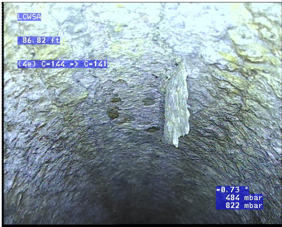
Pictured above and below: 10" ACP sewer main continuing to flake and peel away reducing the structural integrity of pipe (downstream of foremain tie-ins from PS 3E and 4E)
