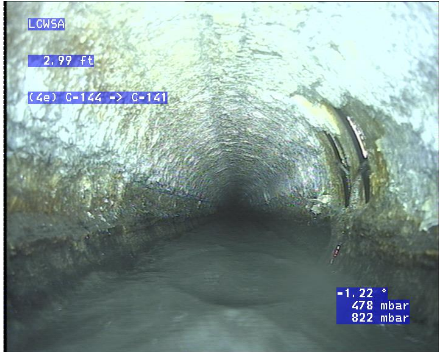
Pictured above and below: 10" ACP Sewer Main downstream of Pump Station 4E with exposed gaskets, creating a high level of infiltration & structural integrity of pipe is approaching failure.
