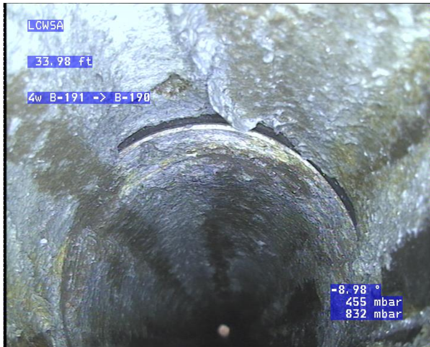
Pictured above and below: 8” ACP Sewer Main downstream of Pump Station 4W with exposed gaskets, creating a high level of infiltration & structural integrity of pipe is approaching failure.
