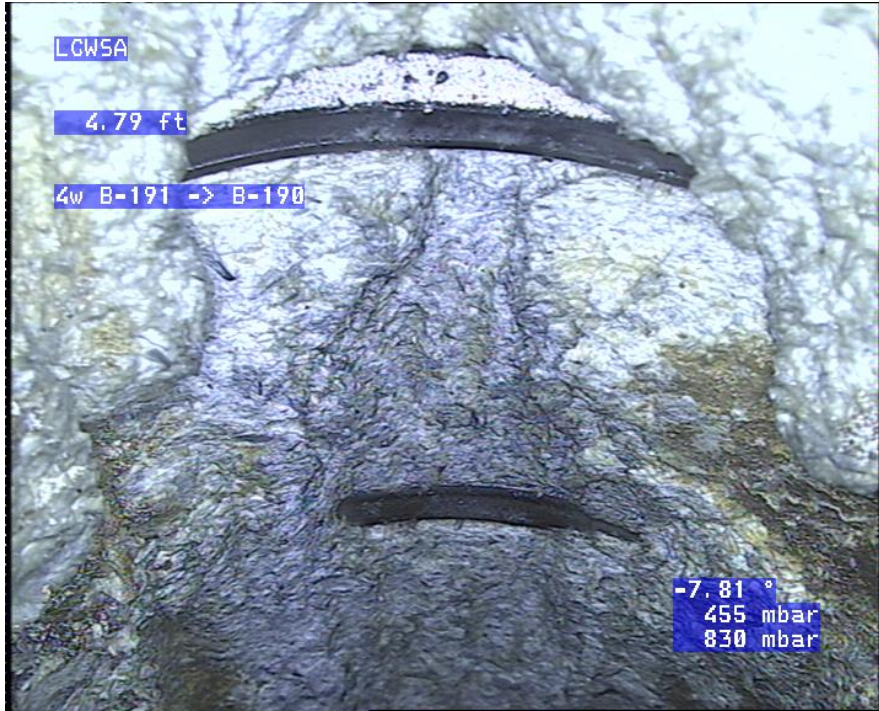
Pictured above and below: 8” ACP Sewer Main downstream of Pump Station 4W with exposed gaskets, creating a high level of infiltration & structural integrity of pipe is approaching failure.
