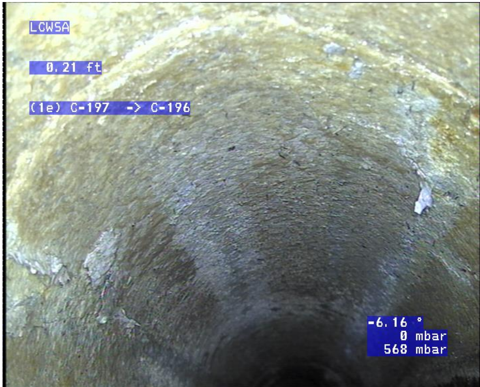
Pictured above and below: more instances of peeling material, spalling and cracking of ACP sewer mains
